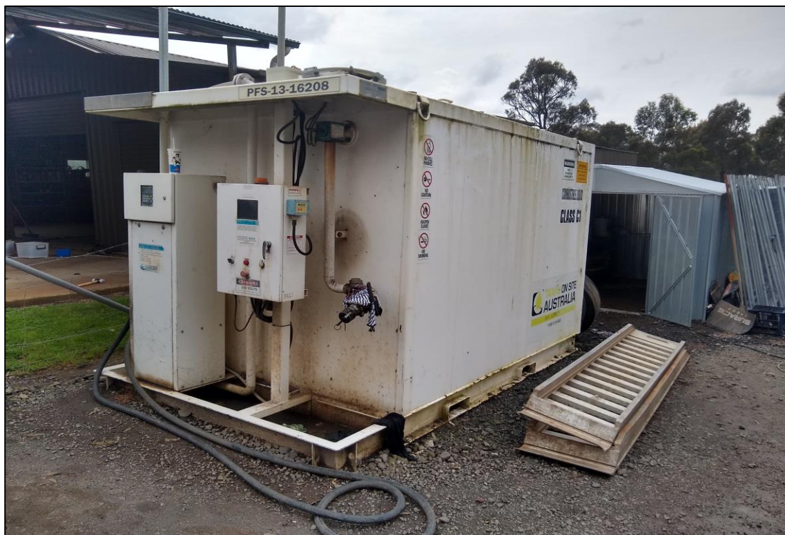
Photograph 17 - A 13,000 L above ground storage tank (AST) used for the storage of diesel was present directly south of the large shed.
