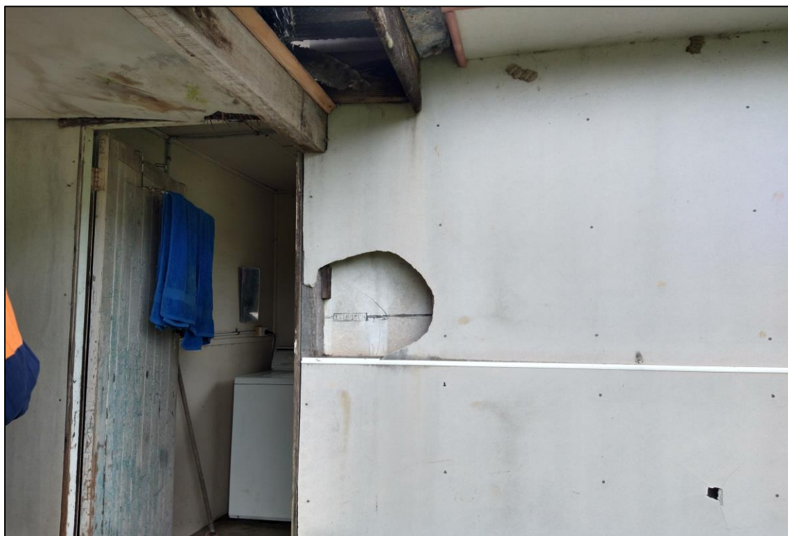
Photograph 2 - 'Hardiflex' fibre material, suspected to contain ACM, used in laundry in south eastern portion of Site A.
