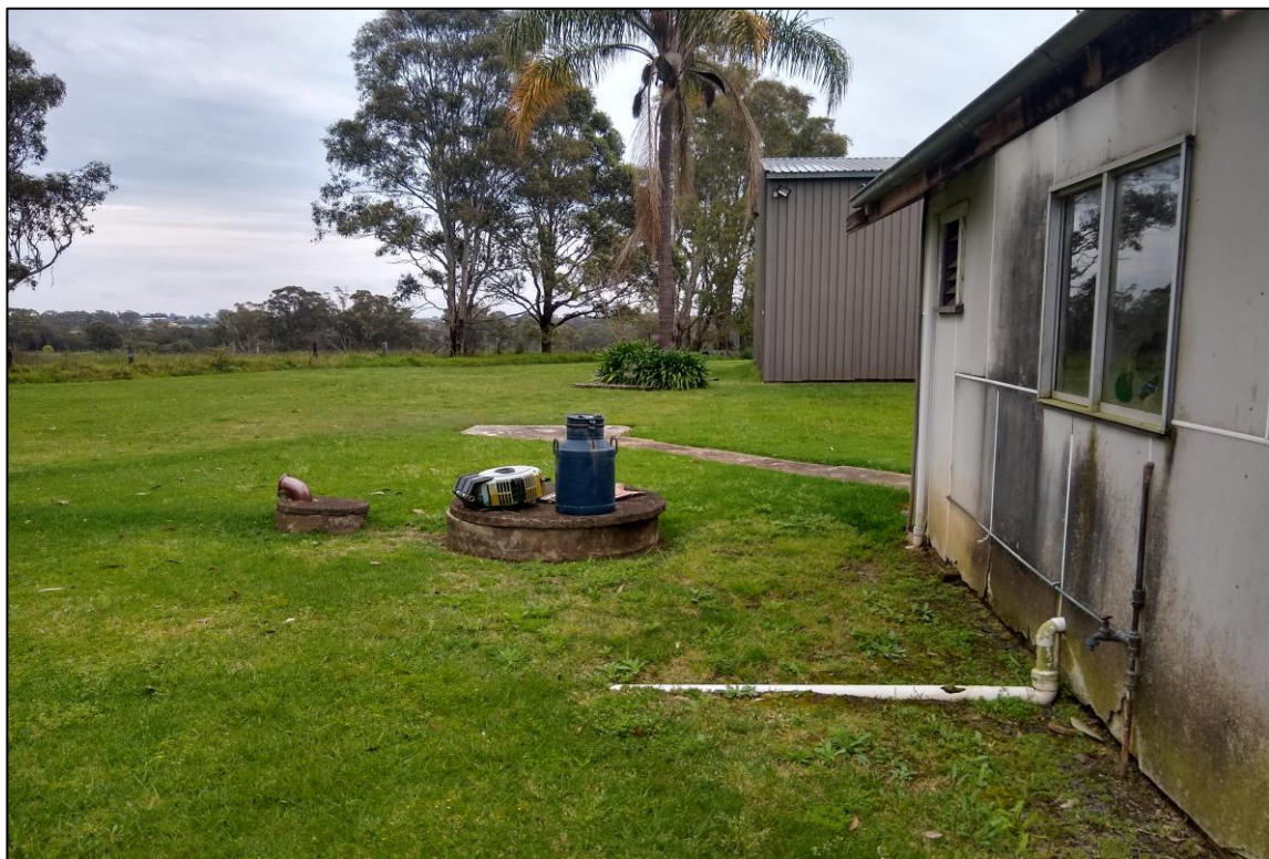
Photograph 6 - Septic tank identified in the south eastern corner of Site A, appearing to be connected to a nearby PVC pipe, which was in poor condition.
